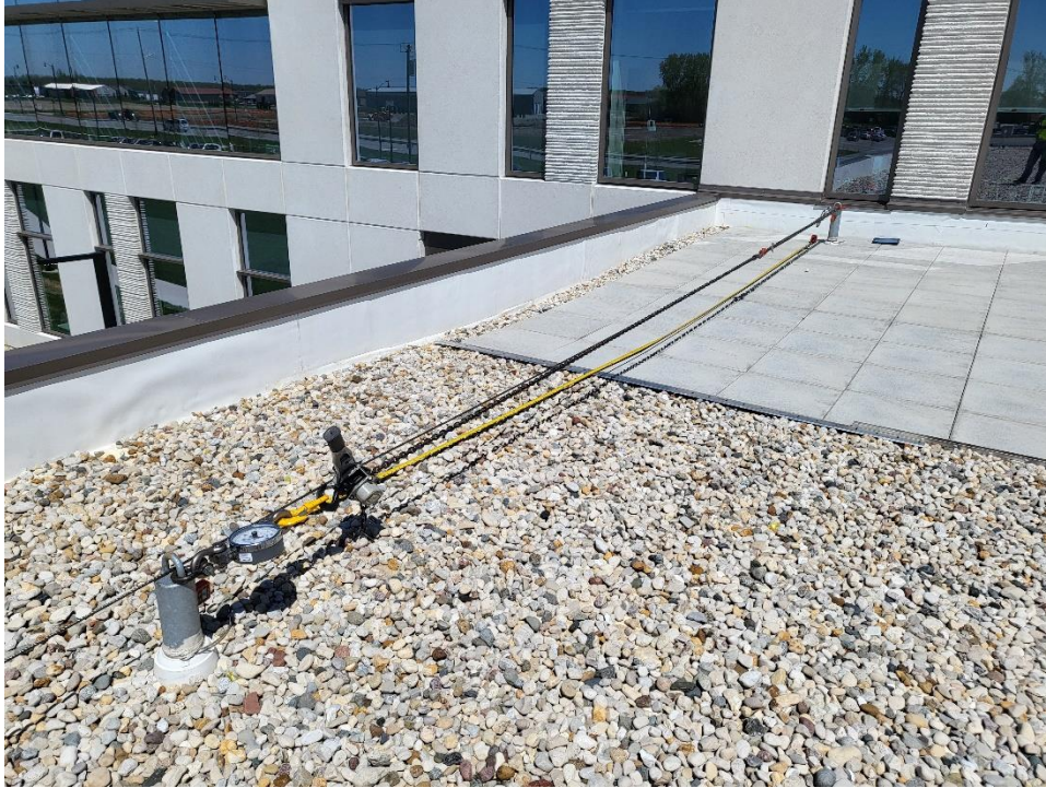
Photo 1 – Load test between 2 tie-back roof anchors (A-11 & A-12).
