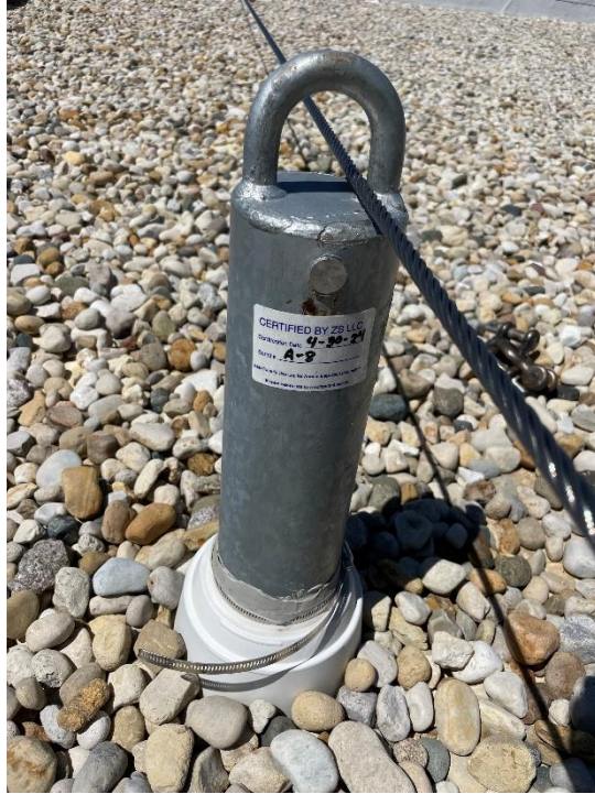
Photo 3 – Certified tie-back roof anchor A-8. Typical.
